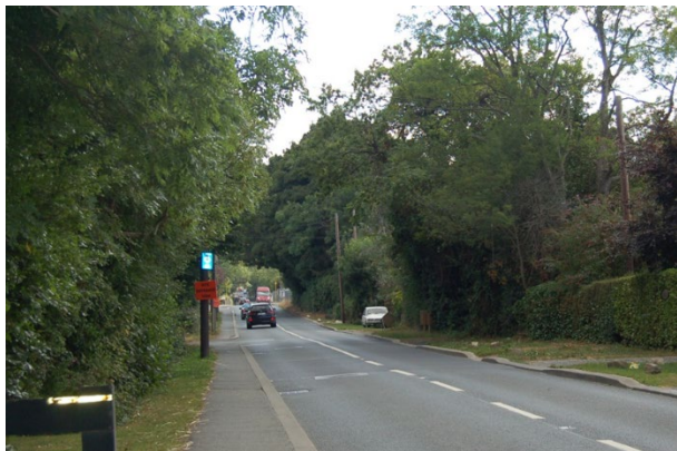
Photograph : Glenamuck Road
