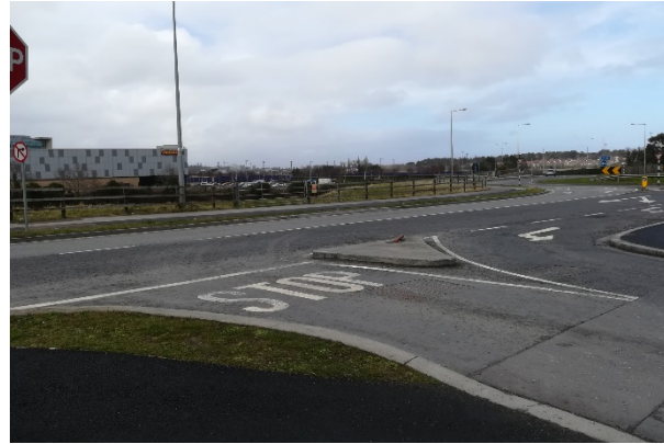
Photograph : Glenamuck Road
