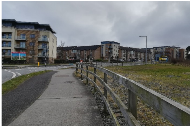
Photograph : Glenamuck Road
